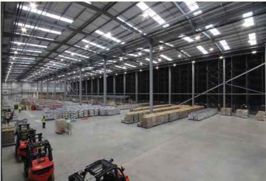
LDH Sproughton Warehouse, an automated warehouse in Ipswich, UK.
