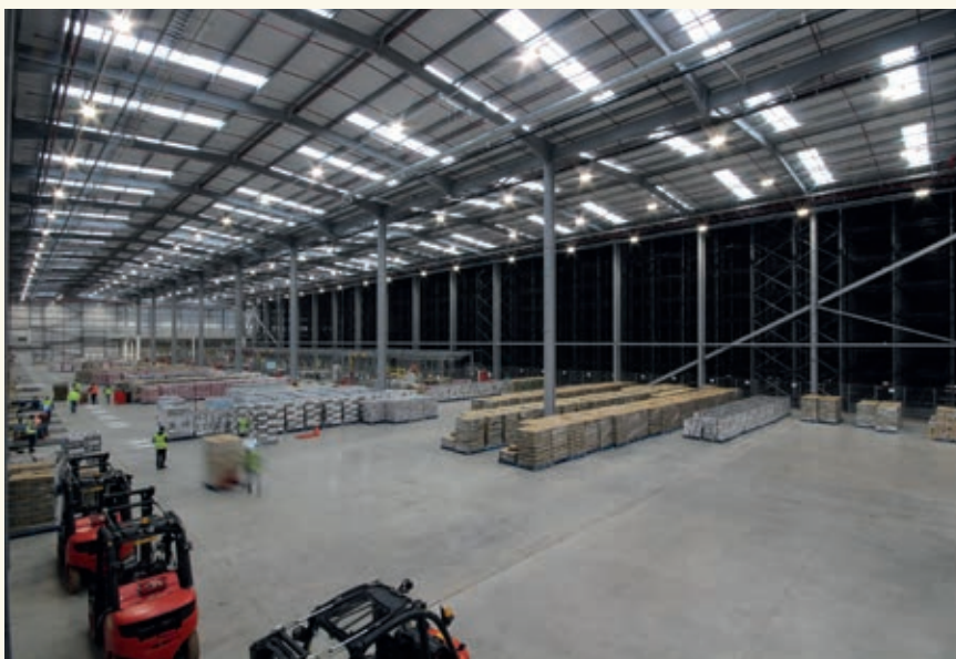
LDH Sproughton Warehouse, an automated warehouse in Ipswich, UK.
